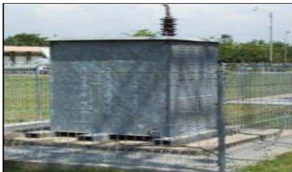
Gambar 2.22 Neutral Grounding Resistance (NGR)
